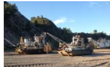
5 x Diesel Pumps
