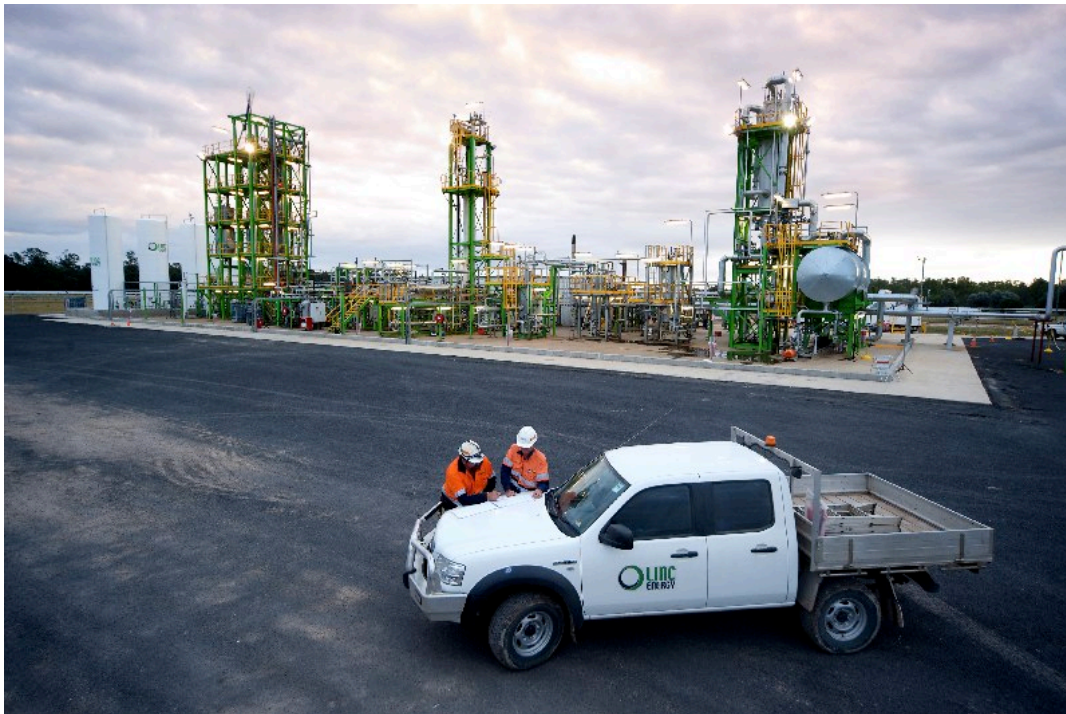
Linc Energy's UCG to GTL Facility at Chinchilla
