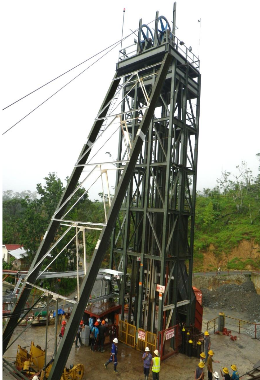
Photo 1: Completed Saga Shaft headframe
