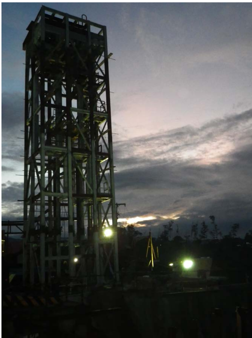
Photo 1: Completed Saga Shaft
