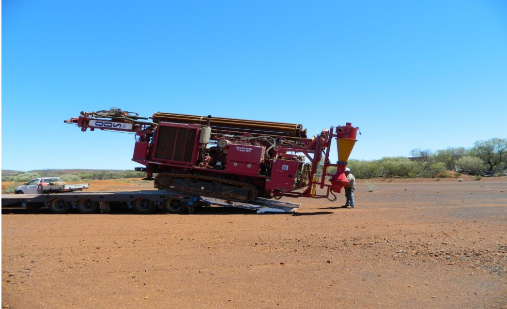
Figure 3: Drill Rig on Site at Gullewa
