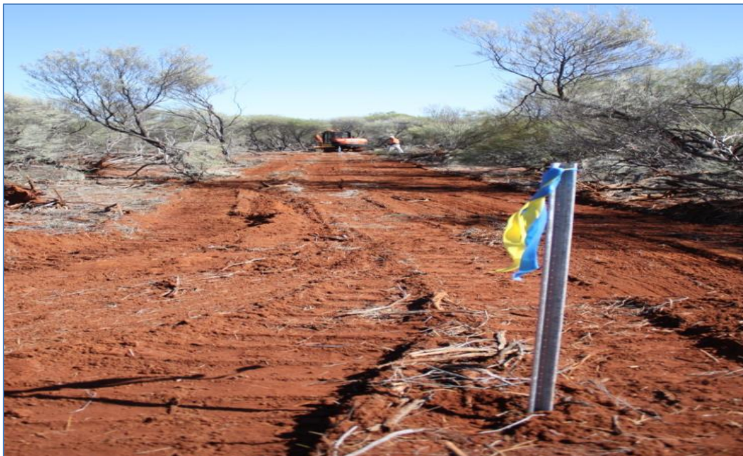
Figure 4: Vegetation and Pad Clearing Activities
