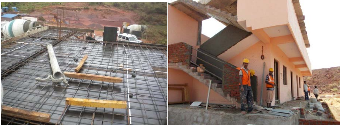
Site Office Construction
