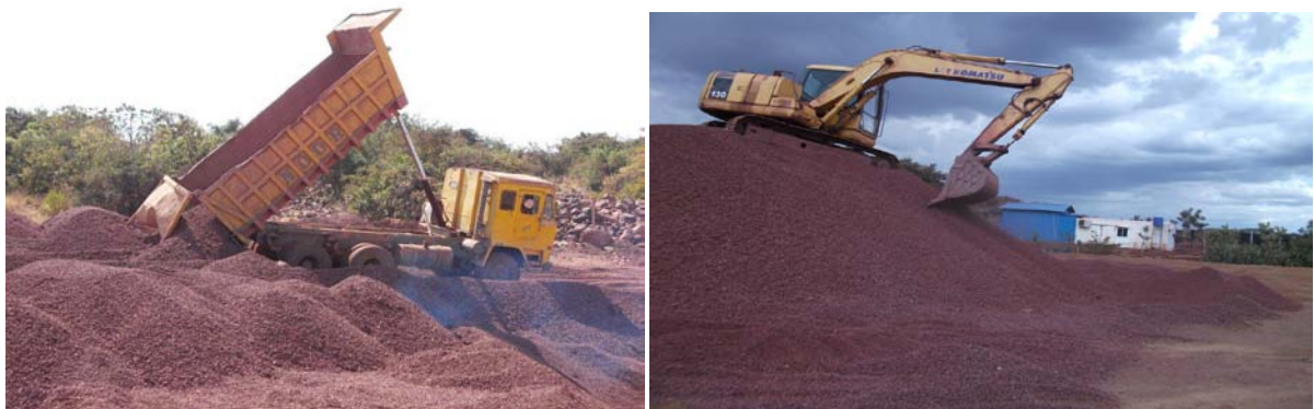
Finished product being stockpiled
