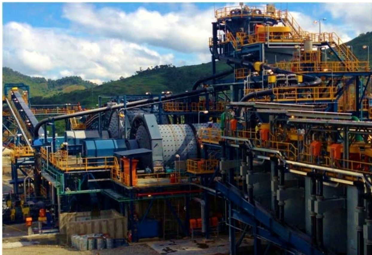
Figure 2: Completed Process Plant, December 2012
