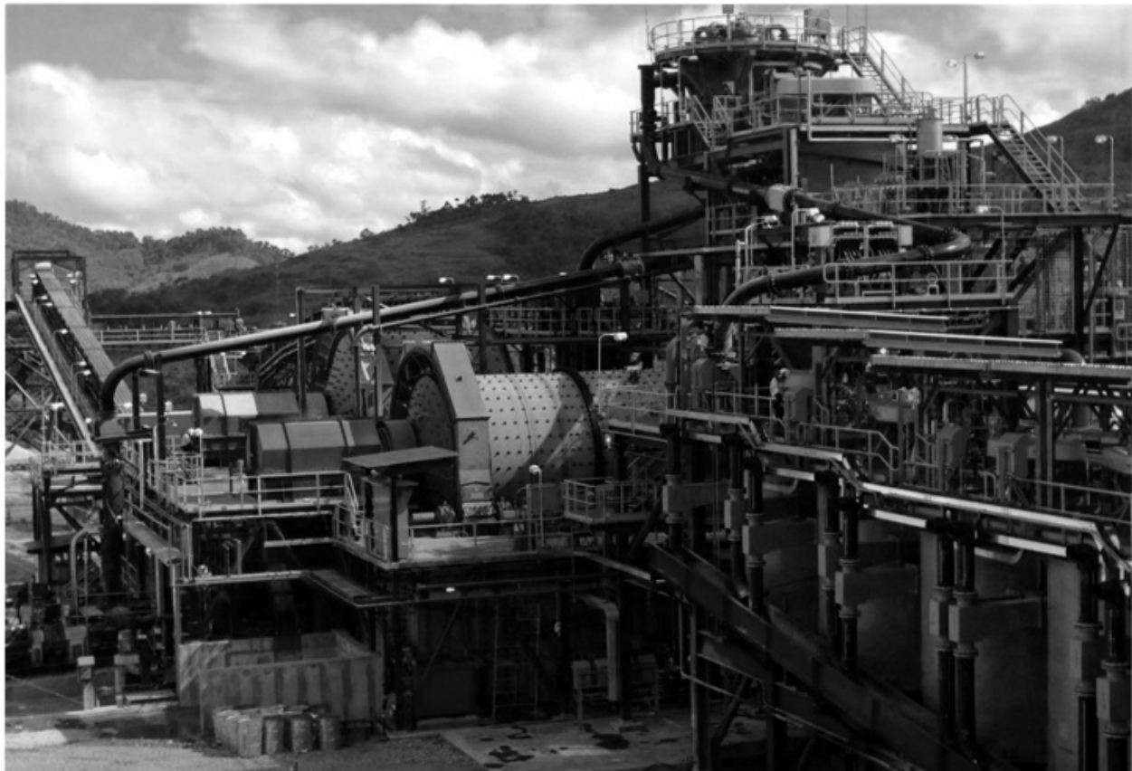
Figure 2: Completed Process Plant, December 2012
