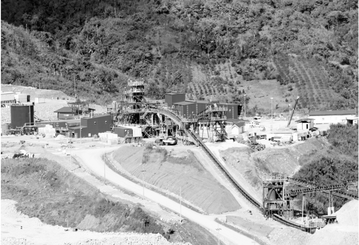
Figure 1: Overview of Process Plant, January 2013
