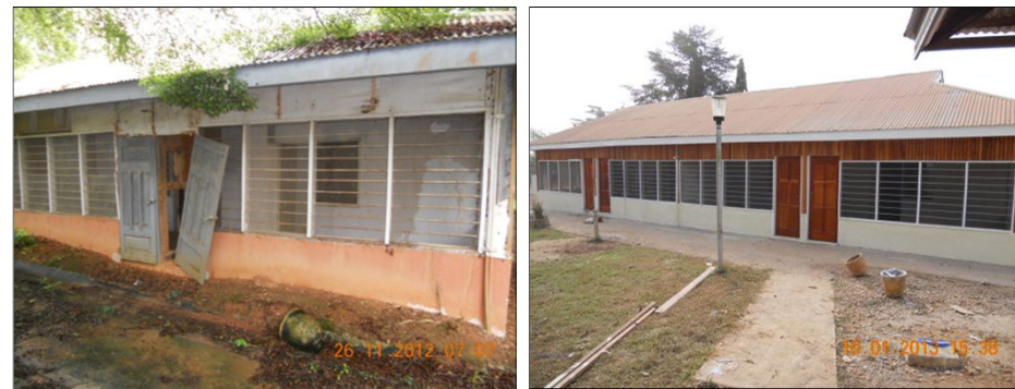
Obotan Camp -Before and After Refurbishment
