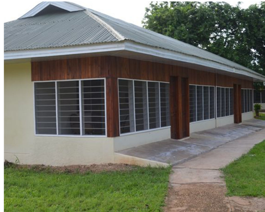
Obotan Camp – After Refurbishment
