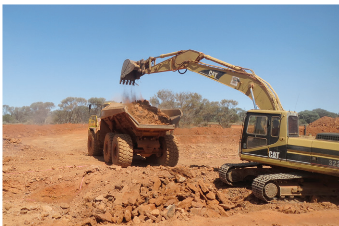
Excavator filling dump truck at Redcliffe Resources 727 Project.
