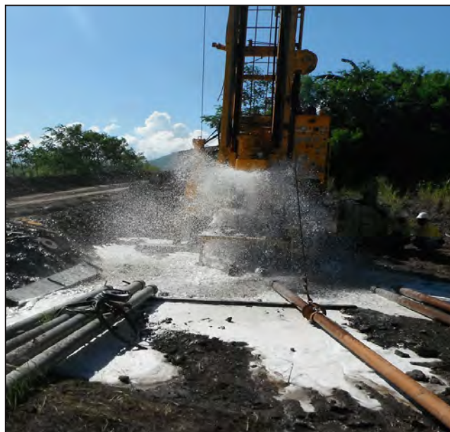
Recent dewatering bore completed 30 March 2013 showing excellent water yield.
