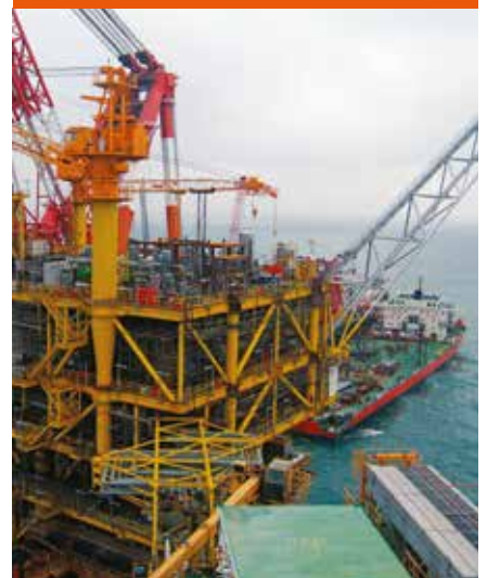
Platform top side installation
