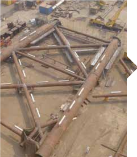
Platform jacket fabrication
