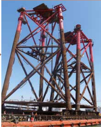
Platform jacket loaded onto barge in preparation for moving to location
