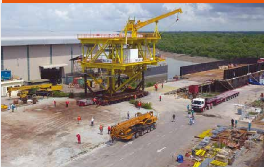
Preparing to load well head platform onto barge for transportation
