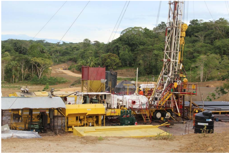
Figure 1: QUN 135 well drilling
