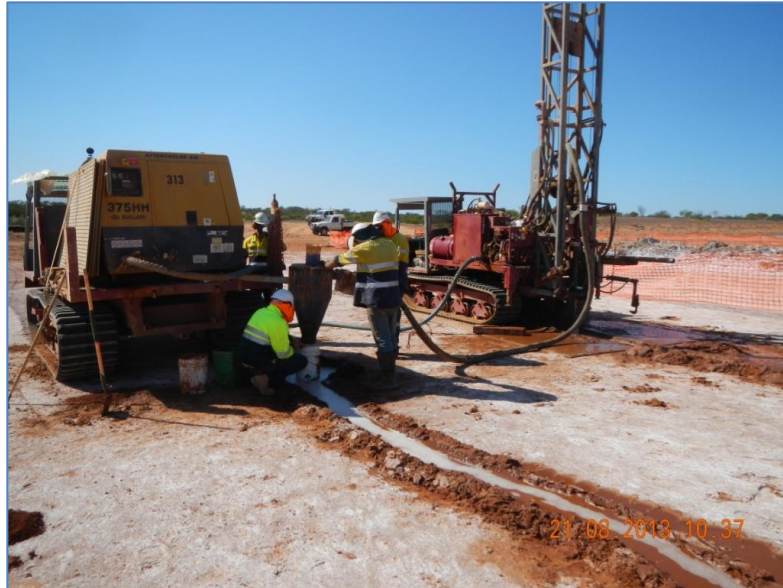
Sampling brine from air core drill hole.
