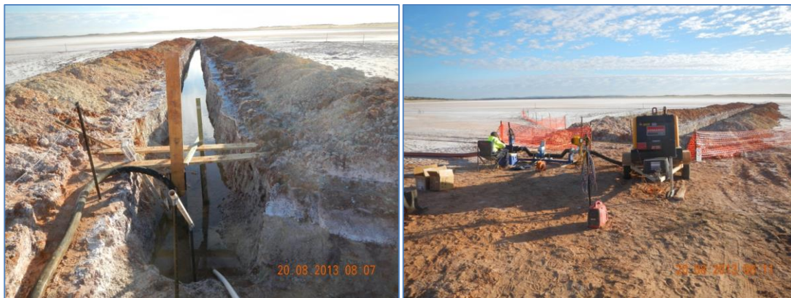
Curtin Boundary Trench with pump testing in progress.
