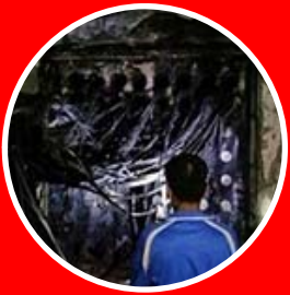
Cable Chamber Operations
