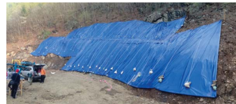
Preparation of diamond drilling pad.
