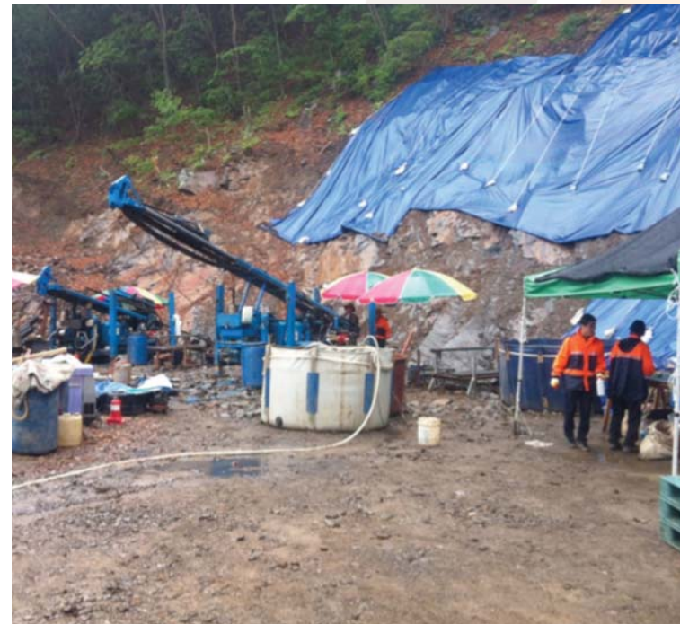
Chubu diamond drilling at Site 1.
