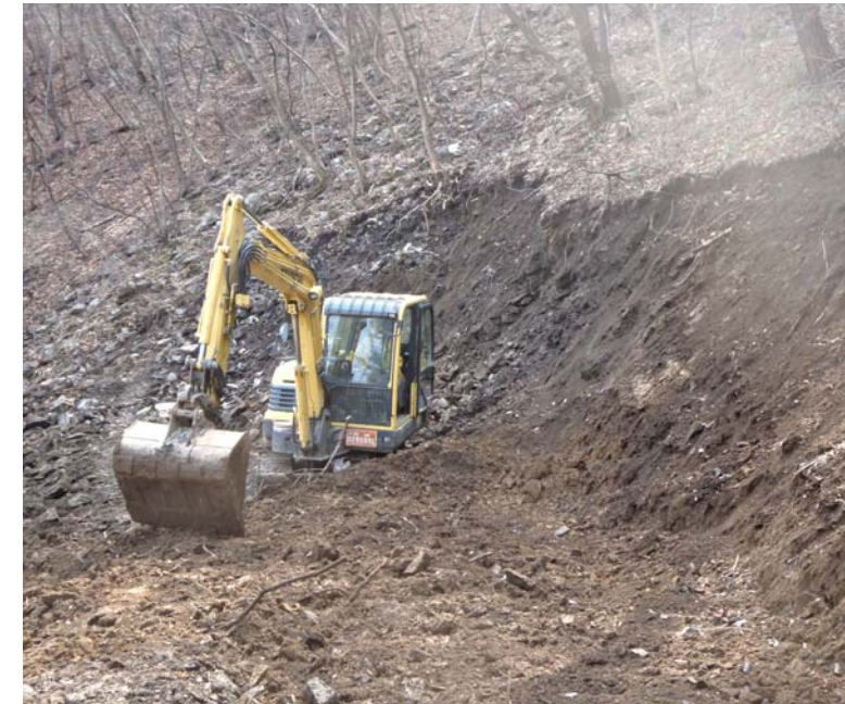
Preparation of diamond drilling pad.
