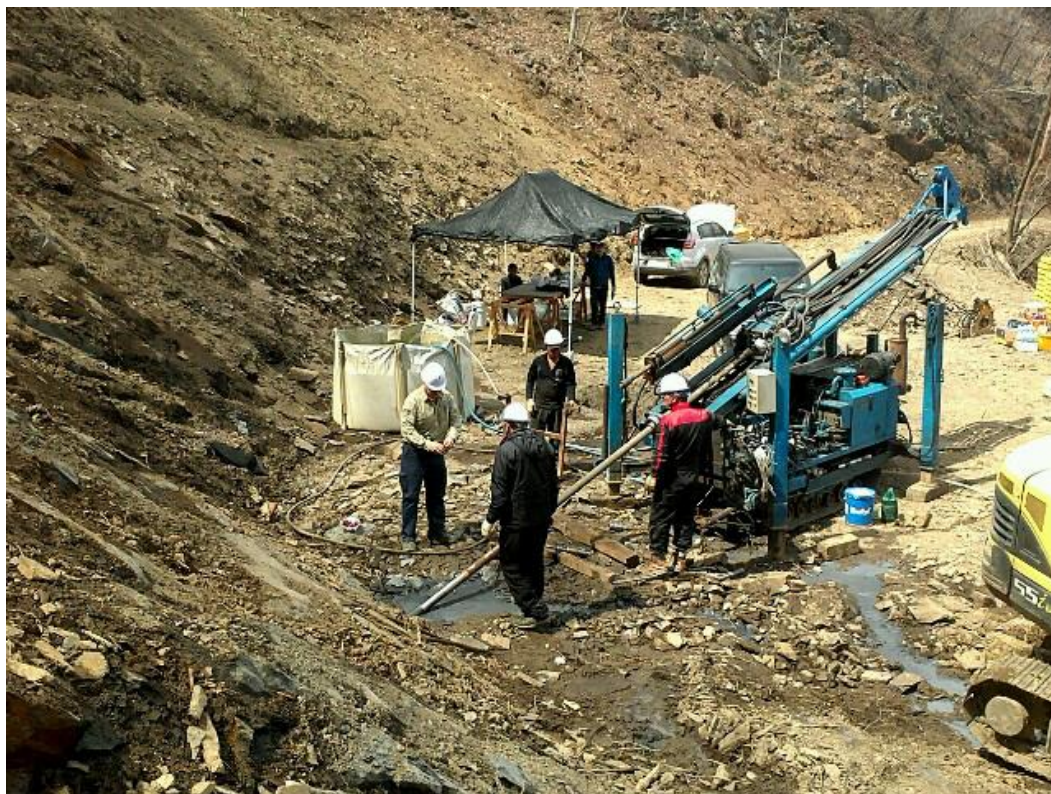
Figure 9: Site 1 and start of Chubu diamond drilling program Thursday, 4 April 2013
