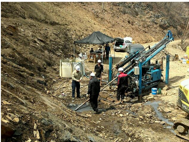
Figure 3: Site 1 and start of Chubu diamond drilling program Thursday, 4 April 2013
