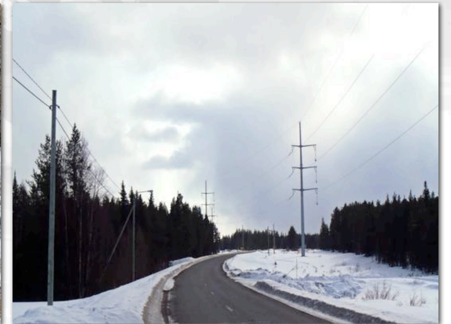
Road and grid power running through project
