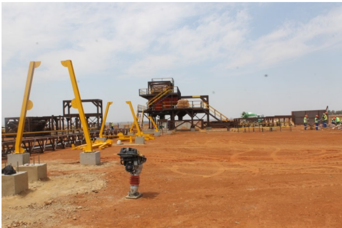
BC1/BC2 secondary crushing and screening module constructed on site
