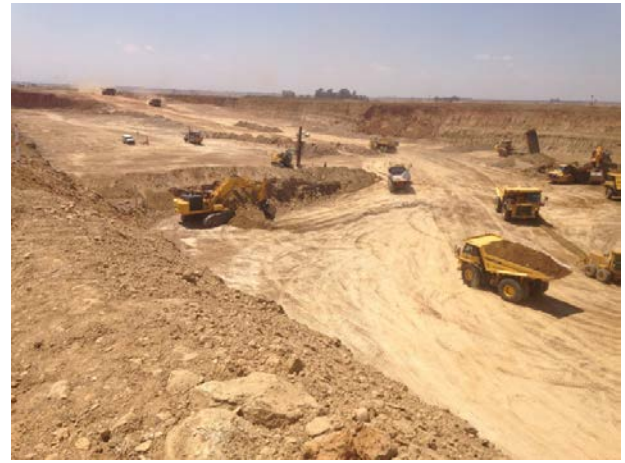
Mining activities in the box-cut
