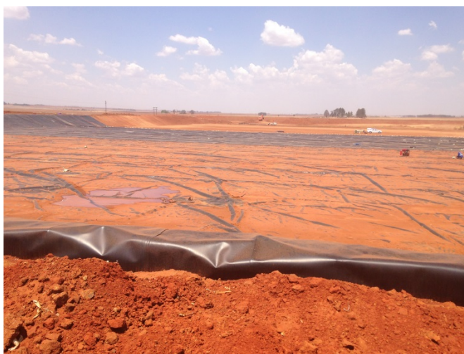
Lining of the pollution control dam underway
