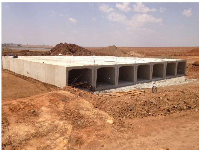
Portals for river crossing installed
