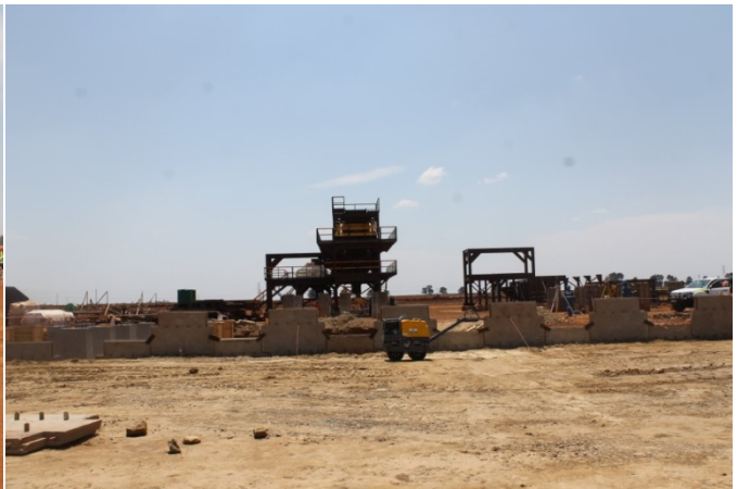
Construction of the plant wing-wall underway
