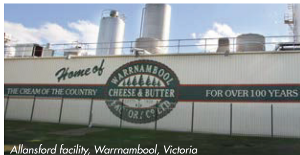
Allansford facility, Warrnambool, Victoria
