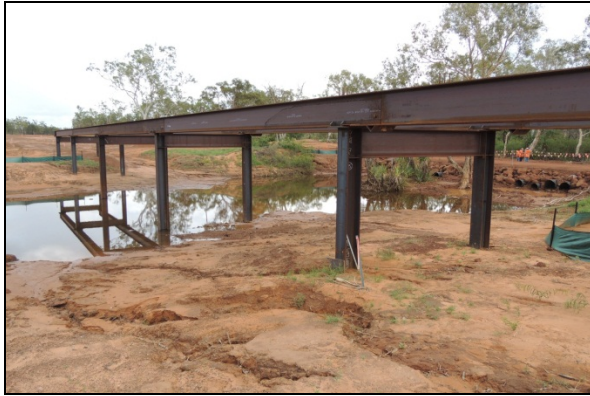
Pine Creek bridge
