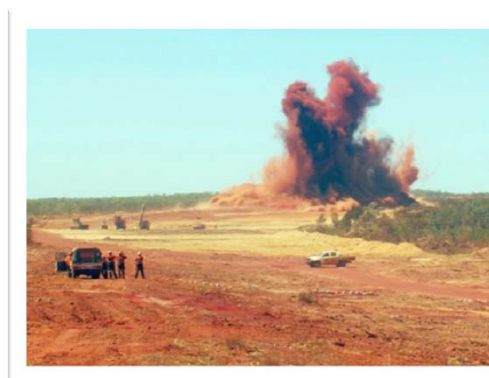
Blasting at Danehill pit
