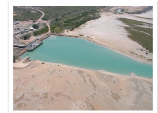
Bing Bong Loading Facility
