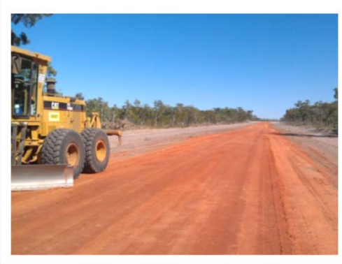
Haul road construction
