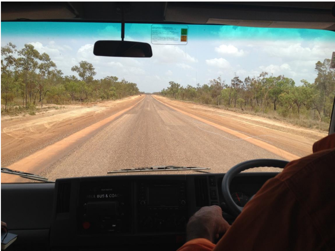
Sealed section of the Haul Road completed in anticipation of production
