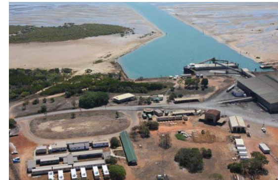
Bing Bong loading facility
