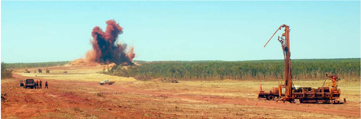
Figure 5. Mining operations at Area F East.
