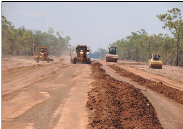
Haul road pavement construction
