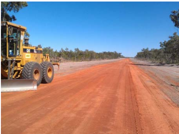
Formation work approx. 60km from minesite
