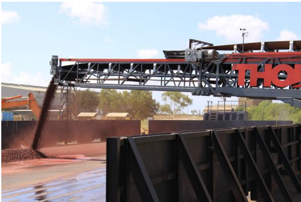
Fig 5: Loading of Barge
