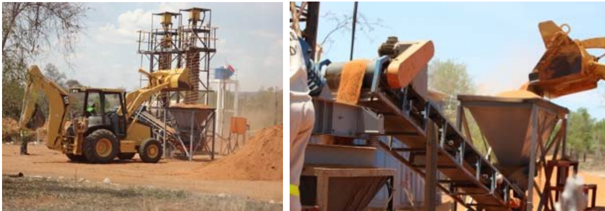
Figure 3 – Pilot plant processing ore from trial mining
