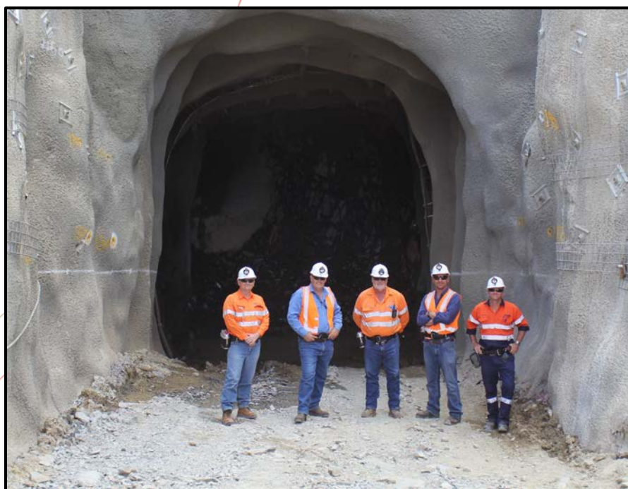
Hera Mine Portal – March 2013
