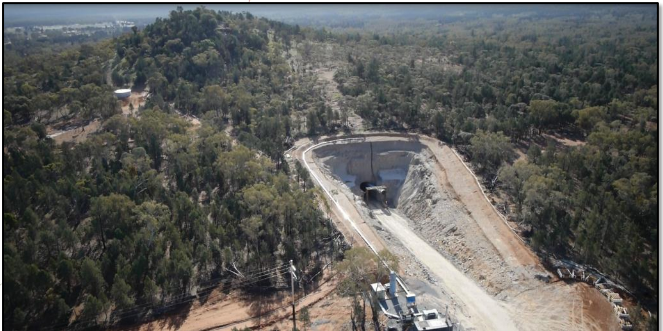
Hera Boxcut and Portal
