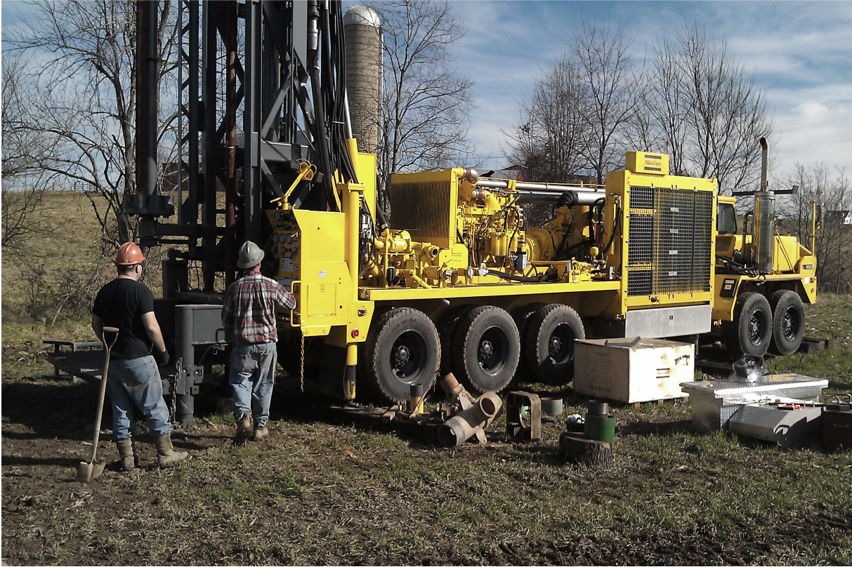
Math Energy RD 20 Range III drilling rig preparing for drilling operations
