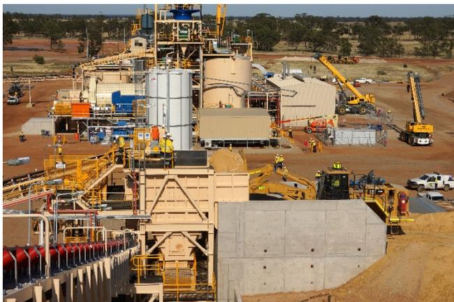
**CIL plant and crushed ore conveyor**
