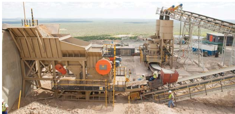
Figure 3: Example of a modular crushing plant
