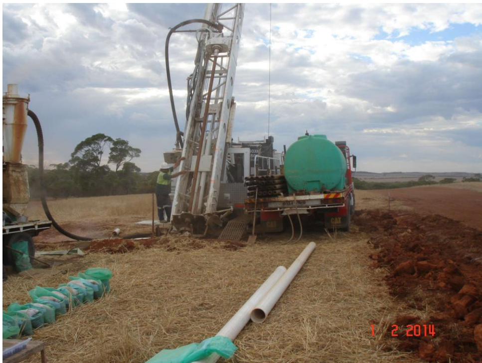
Plate 1. EPIRC14_002 drilling in progress
