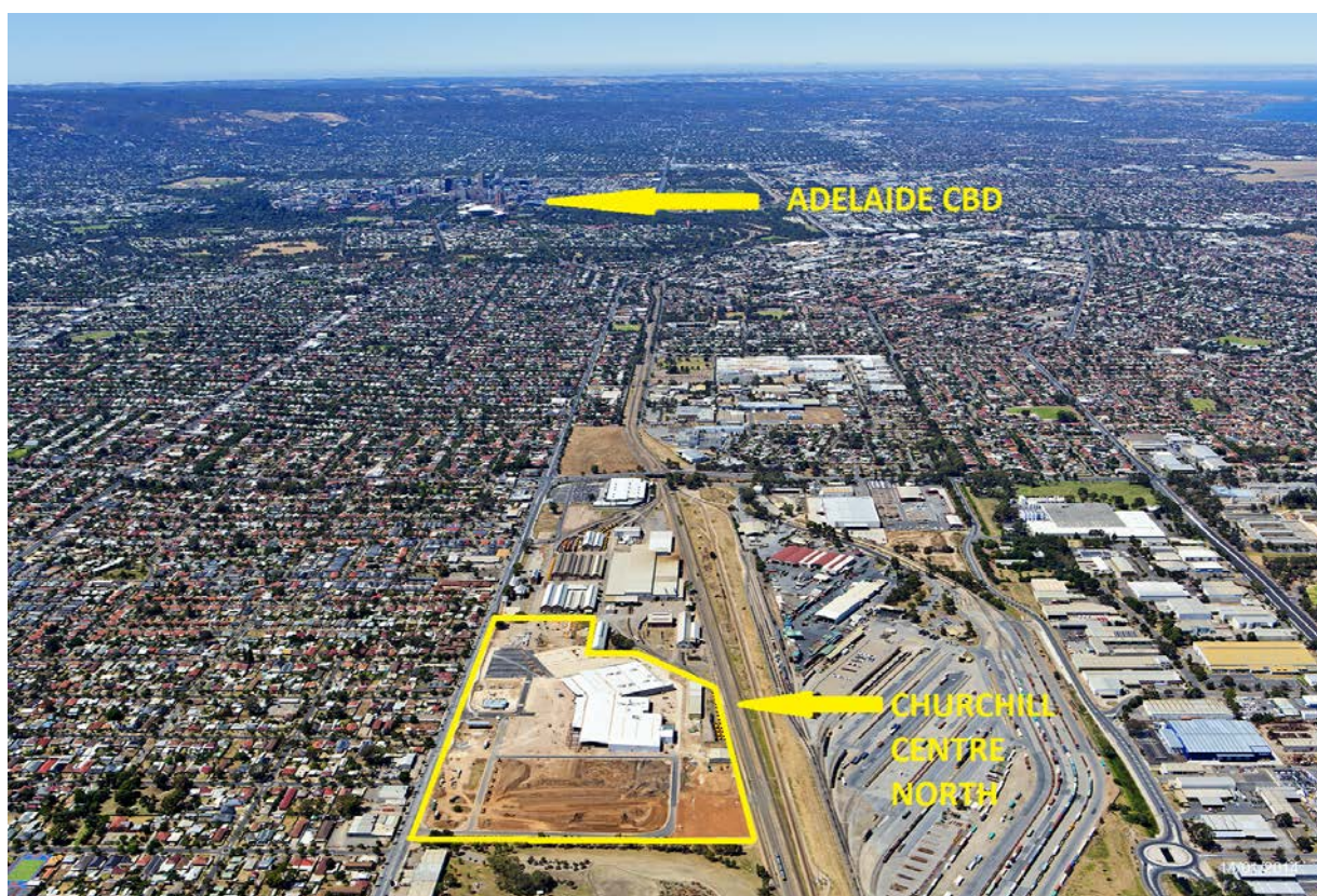
Construction and site earthworks as at 14 January 2014
