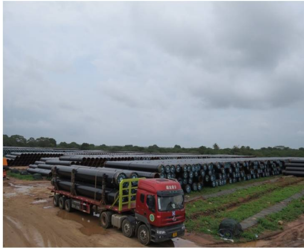
East Tanzania Pipeline project - main 36" pipeline lay down area.
