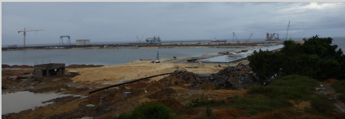
Kribi deep water port nearing completion October 2013, on target for 2014 opening
