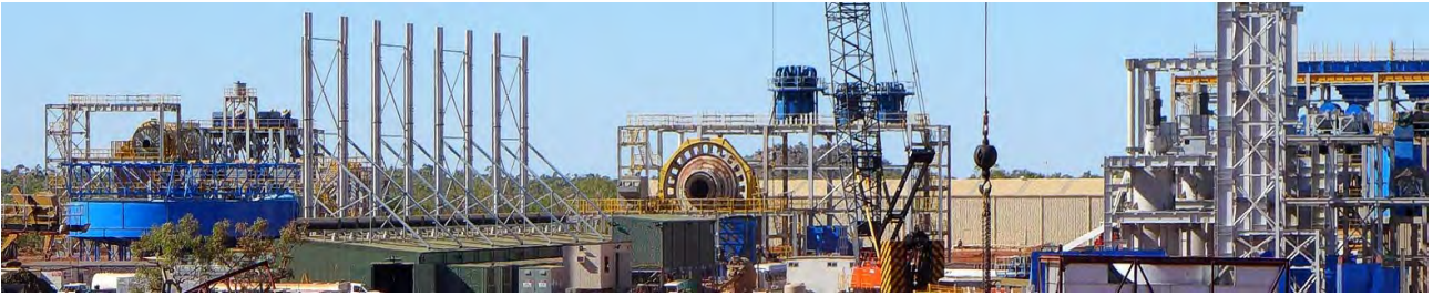
Figure 17 (left to right): Gravity Thickener (blue tank) and Scrubber (behind), power station with exhaust stacks, Ball Mill, Flotation Cell building behind re-grind circuit.
