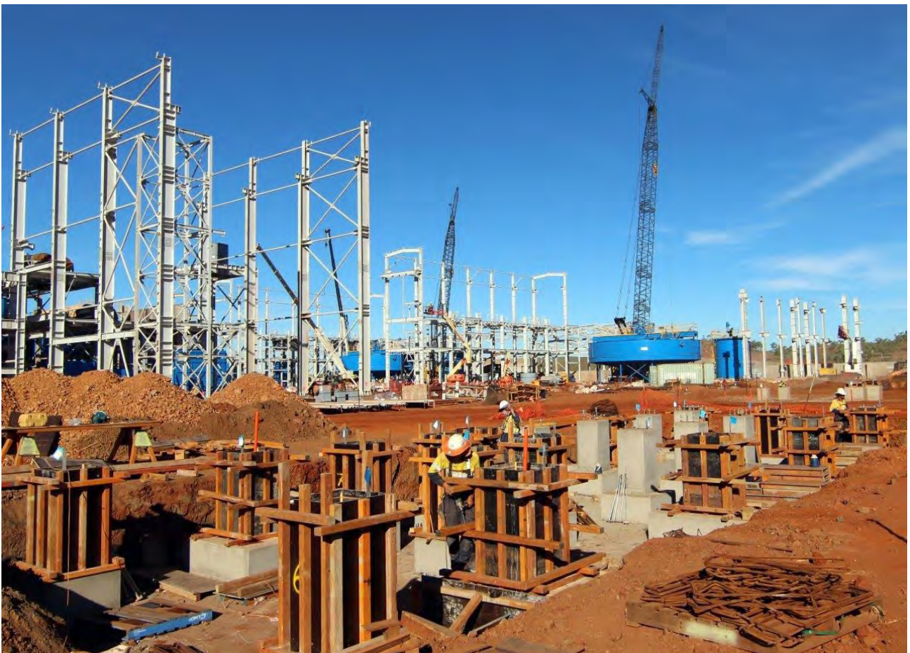
Figure 23: Flotation Reagents Building footings ready for the final concrete pour
