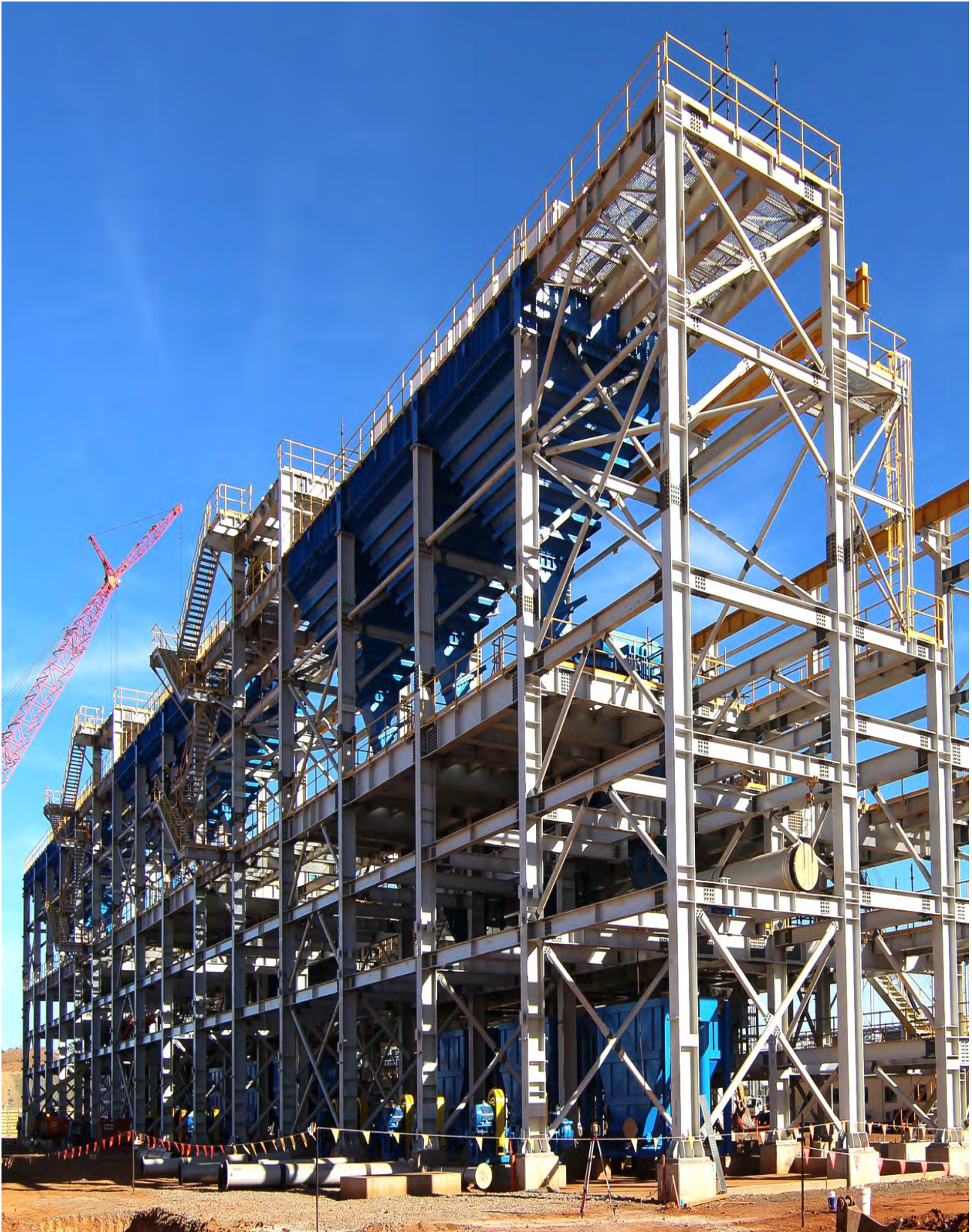
Figure 21: Gravity Jig Building - top floor sections now in place
