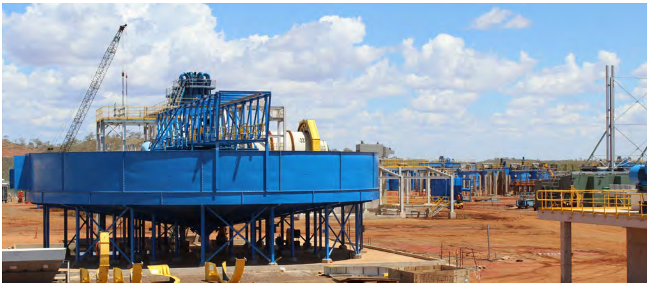
Figure 16: Gravity Thickener with Ball Mill in background
