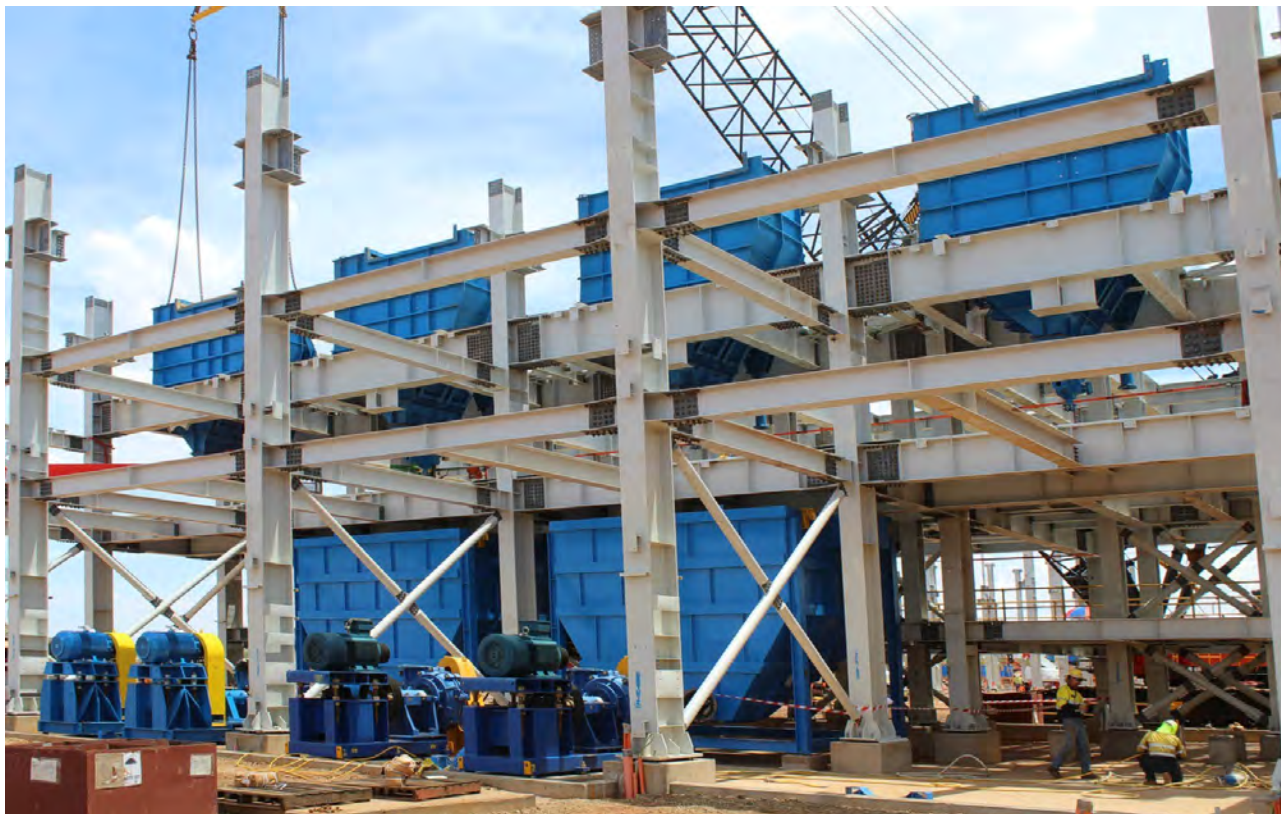
Figure 29: Gravity Jig Building - capable of processing 3mtpa and is the largest continuous gravity jig in the world.
