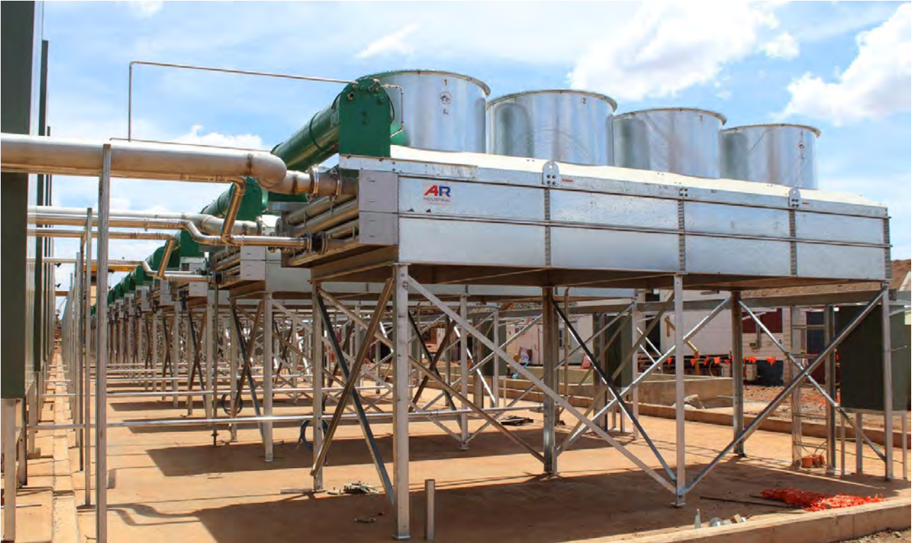
Figure 25: Cummins Power Station cooling system
