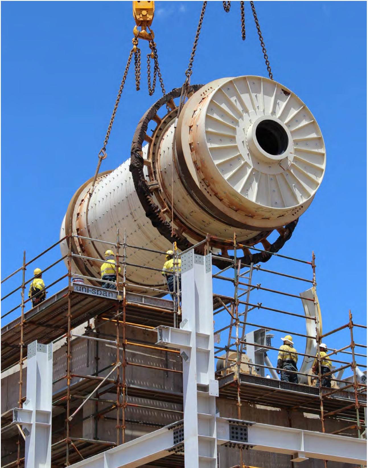
Figure 4: Scrubber (de-agglomerator) recently lifted into place.
