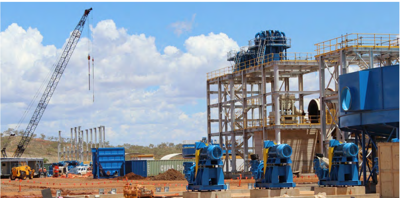
Figure 24: Gravity Thickener (foreground) and Ball Mill in the Background
