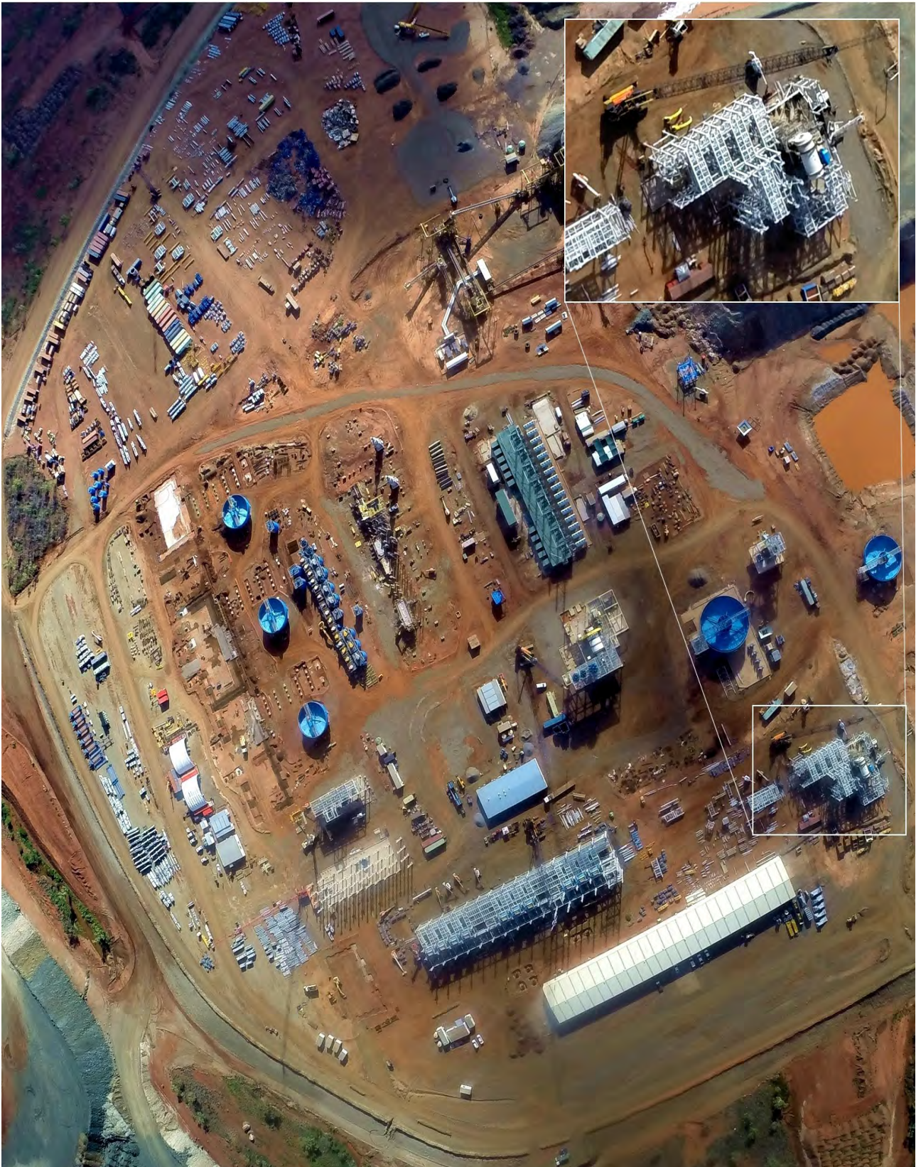
Figure 5: Process Plant taking shape - Scrubber highlighted
