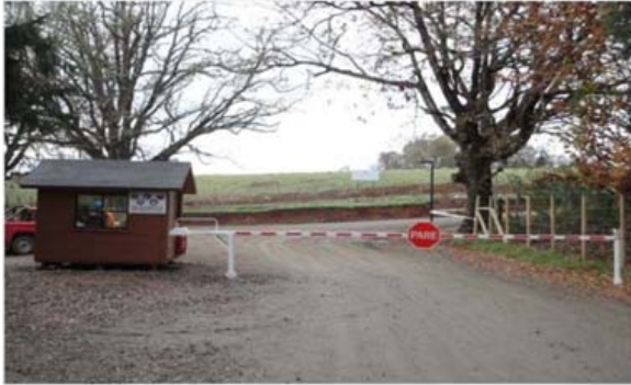
Site Established - Entrance
