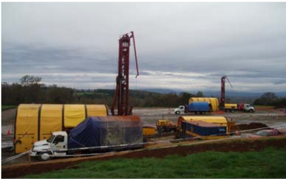
Monitoring Well Drilling on Vertical Drilling Pad
