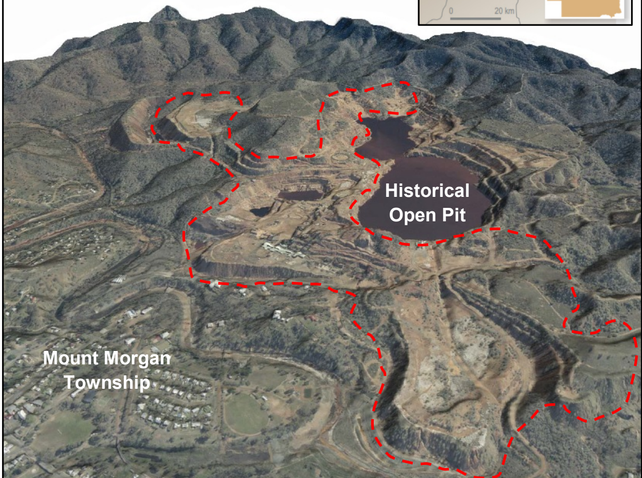
Figure 3: Site overview of the Mount Morgan Mine
