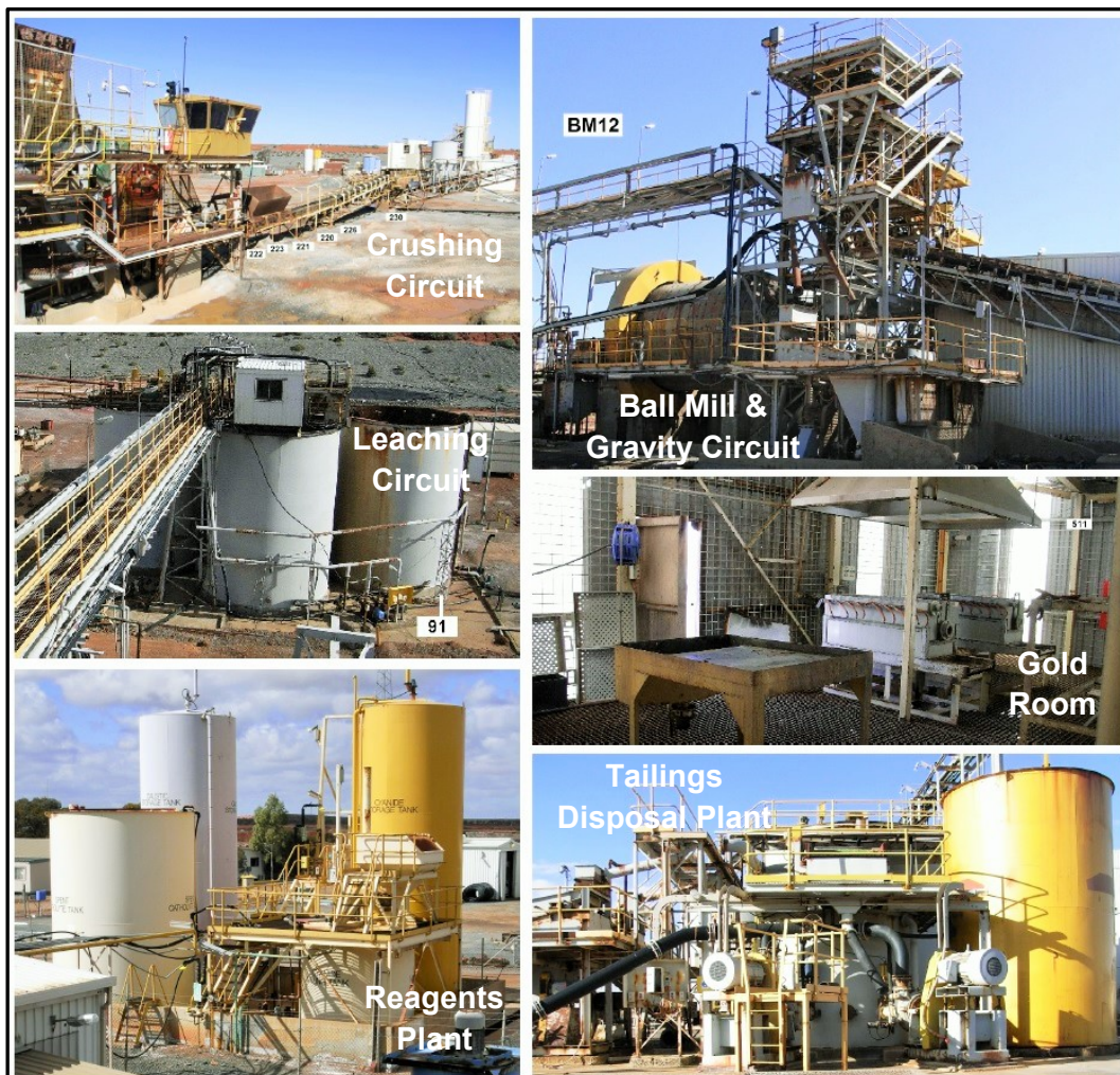
Figure 4: Kundana CIP Plant (pre-decommissioning and refurbishment)
