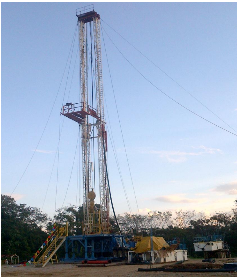
Rigged up on Atzam #5 location
