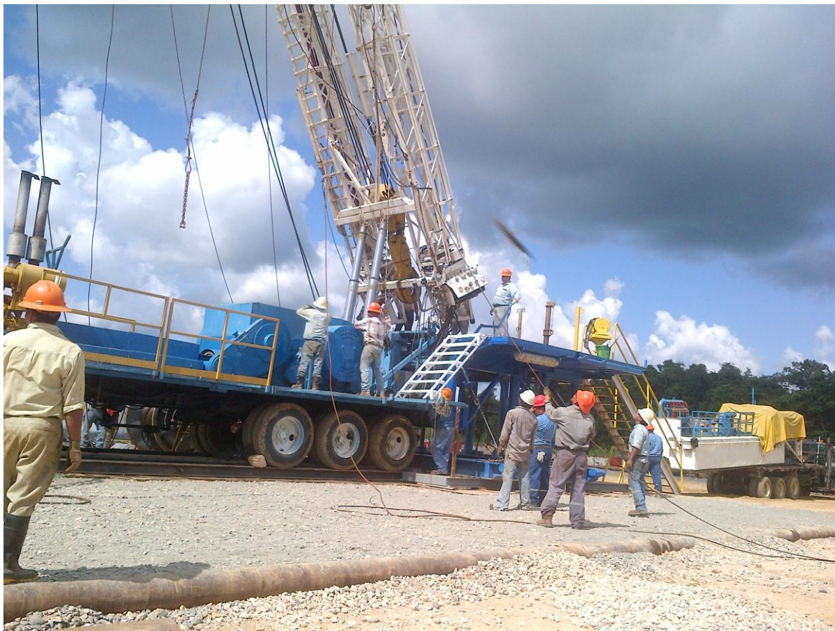
Rigging up mast on Atzam #5 location
