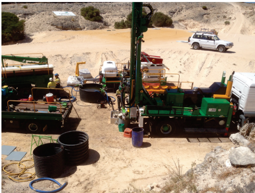
Seawater intake bore being drilled, Garden Island, WA
