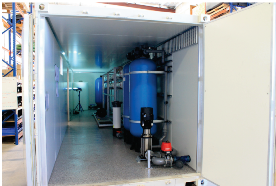
Containerised desalination plant being assembled
