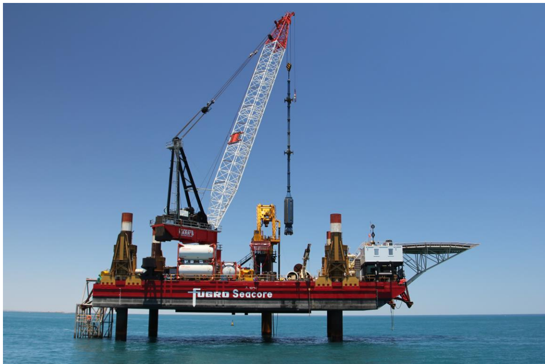
Offshore foundation works at Garden Island, Western Australia
