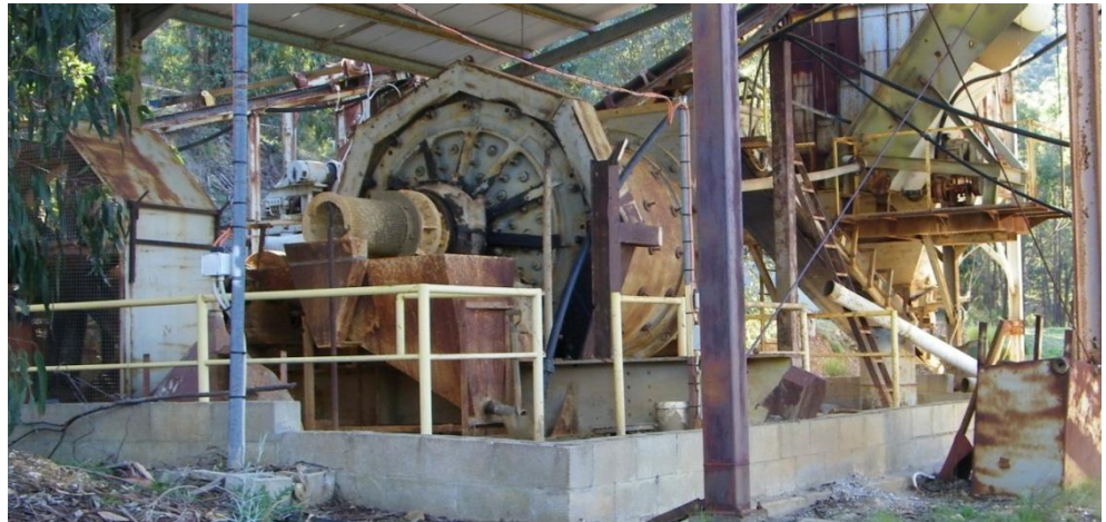
Fiddlers Creek Ball Mill has replaced Ball Mill No1 at Inglewood
