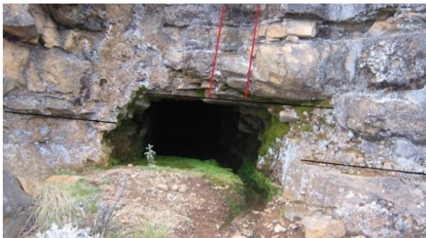
Figure 6: Historic mine entrances ("adits") at Chanape. The vein systems (orientation shown with red lines) are sub-vertical. There are more than a dozen such adits in the Chanape Project area.
