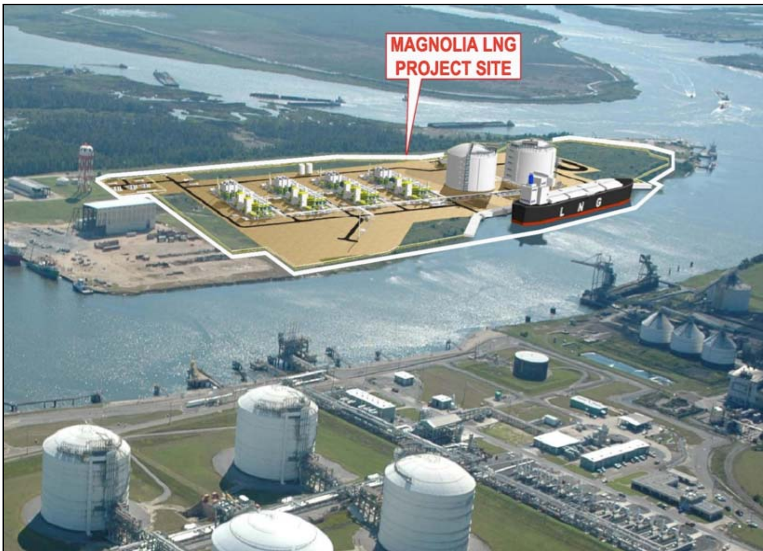
Figure 1 – Schematic Representation of the Proposed Magnolia LNG Project at the Port of Lake Charles, Louisiana, US
