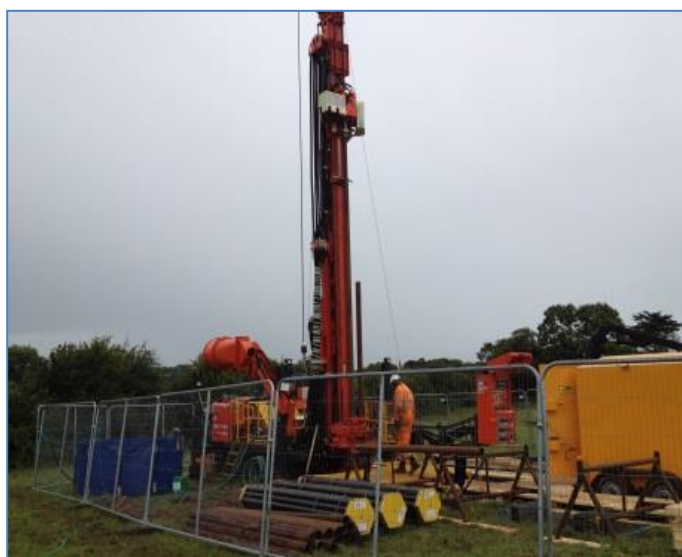
Figure 1 Priority Drilling Operating the Hanjin D&B35 Rig
